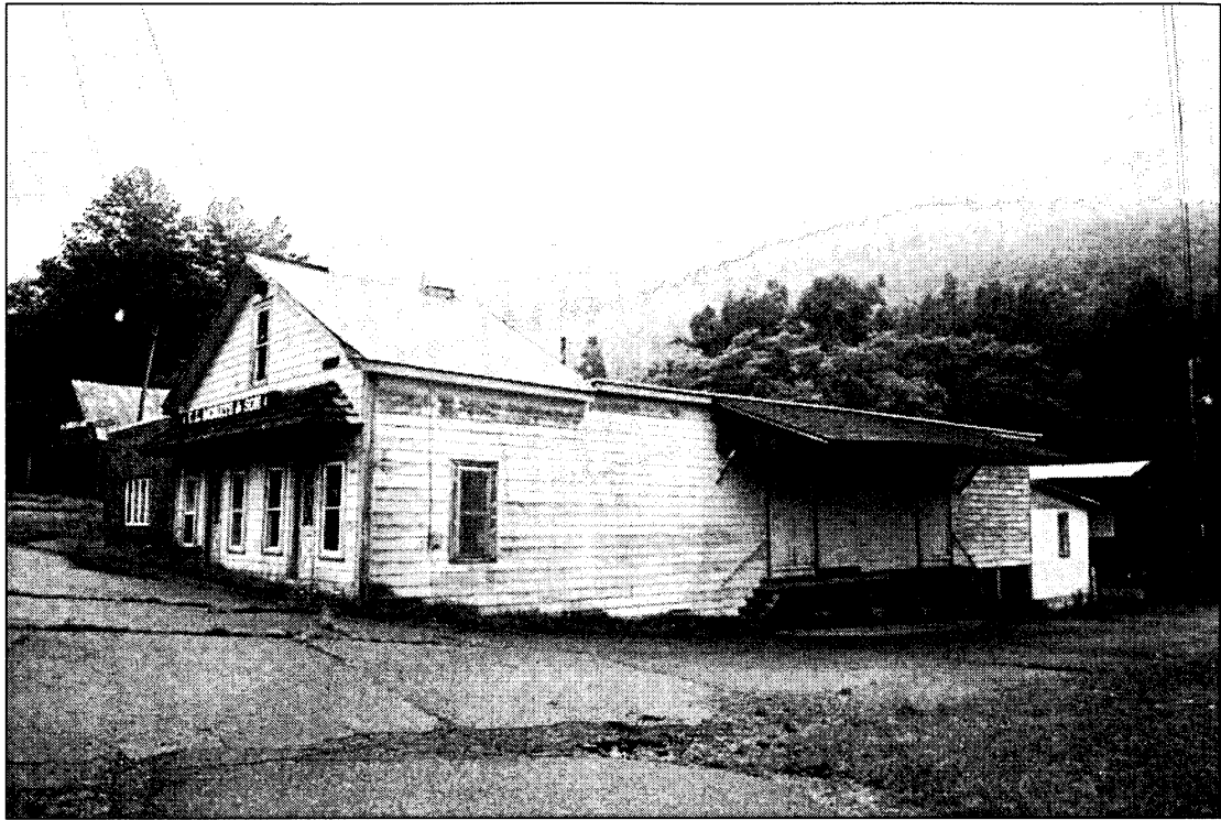
Office and store, looking south.
