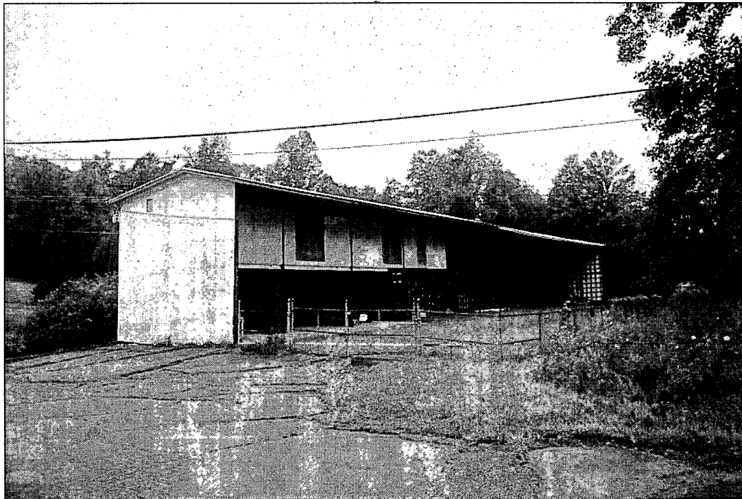
Lumber shed, western side of complex across drive, looking southwest.
